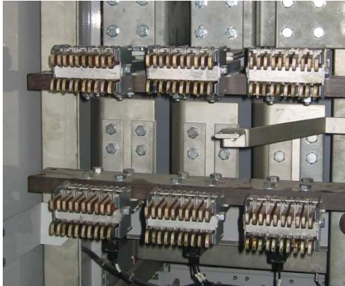
Old cluster contacts and springs shown with chassis removed for clarity.
