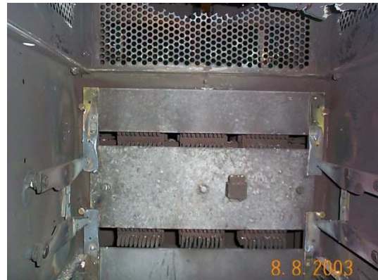
You don't want your ACB cassette to end up like this after a plug-in retro-fit ACB.....
