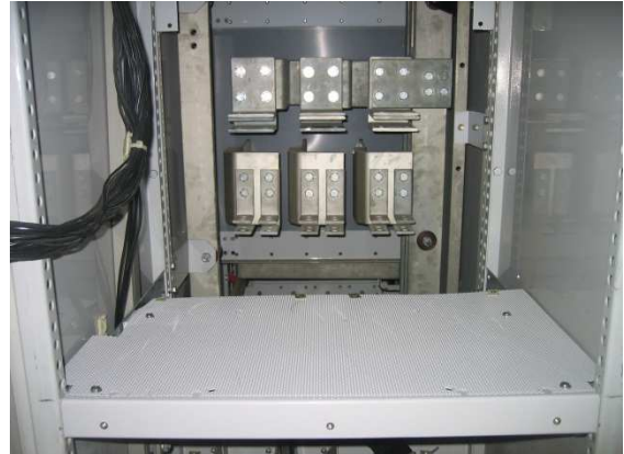
Old cluster contacts and springs shown with chassis removed for clarity.
